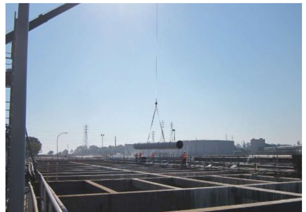
New pipe sections are loaded from the land-based barge to the scaffold work deck.
