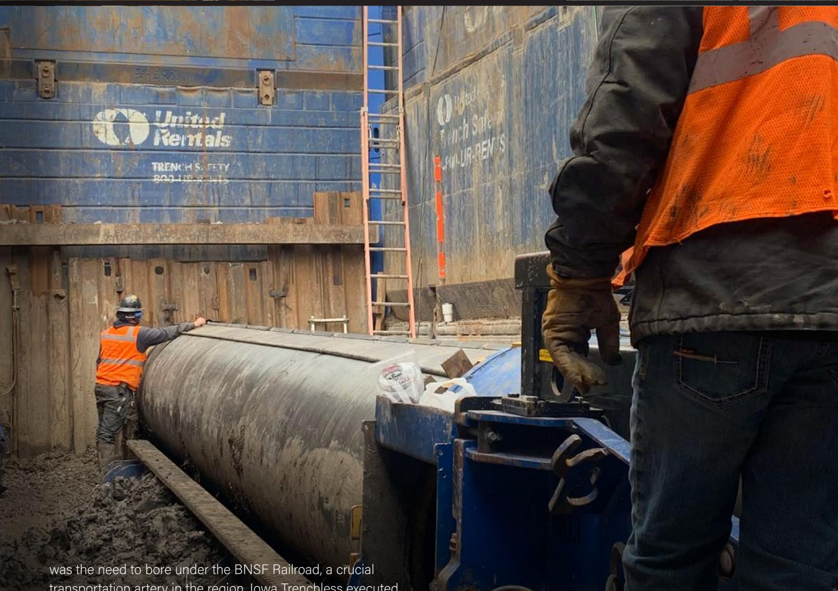
was the need to bore under the BNSF Railroad, a crucial transportation artery in the region. Iowa Trenchless executed this with precision, utilizing an Akkerman Guided Boring Machine and Michael Bryne Auger Boring Machine to install the 140-foot long casing ranging from 32 to 54 inches in diameter for a sanitary sewer line.
