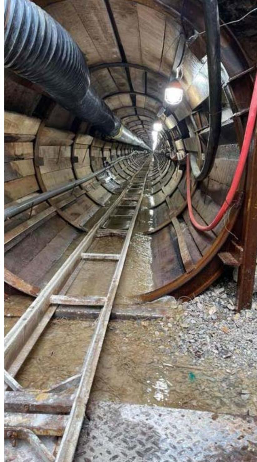
lagging as the tunnel liner, with sets built behind the TBM and then expanded. The decision to select this segmented tunnel lining approach significantly reduced the jacking forces required for the 1,300-ft crossing, as well as aiding in steering the TBM since it is advanced off the installed liner immediately behind.
