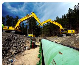
**June Winner: Gavin Felder** When the Thunder Rolls, the Hammer Strikes. Making an impact with TT Technologies Goliath pneumatic hammer - installing more than 130 ft of 42 in pipe in rocky ground. Black Hills, SD Pipe Ramming Job
