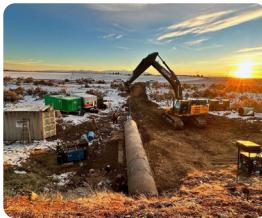
**February Winner: Jon Kile & Joe James** Jon's crew completed this project in Minidoka, Idaho, where a challenging 48" rock bore for the Union Pacific Railroad resulted in successful installation of 140' of 54" steel casing with the Taurus, one of several TT Technologies pipe hammers in our Iowa Trenchless fleet.
