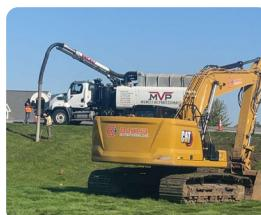
**May MVP Runner Up: Bud Durnan** MVP working with Baker Enterprises in Pella, IA using Hydro-Excavating to locate utilities in preparation for Iowa Trenchless to come in to complete a bore.
