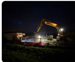
**May Winner: Brandon Derry** Taken on the late nights of the Thornton, CO 104th street crossing project. The crew completed this 140 LF of 54in steel casing utilizing the Pilot Tube Pipe Ramming method.
